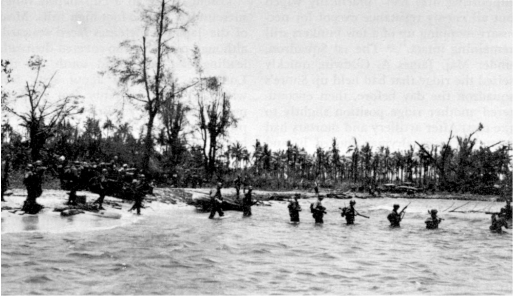
CROSSING THE LORENGAU RIVER over the sandbar at the mouth of the river, 18 March 1944.
